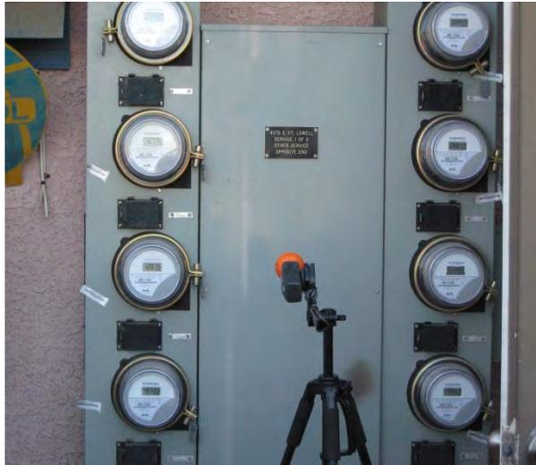
Figure 3. TM-195 placement at a bank of meters.
